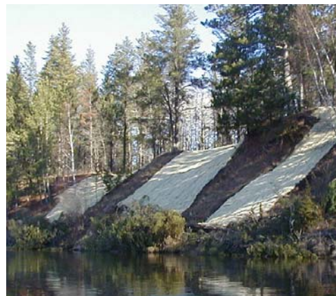
Critical Area Stabilization
