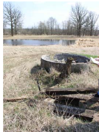
Unused Well Sealing
