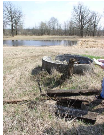
Unused well sealing
