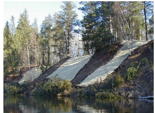
Critical Area Stabilization
